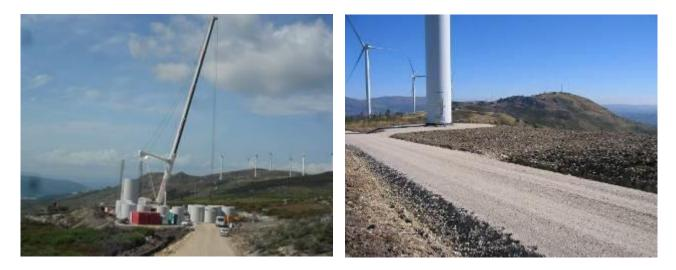
Photographs 4.5 and 4.6 - Example of working platform adjacent to a wind turbine, on the left during the assembly phase and on the right after landscaping
