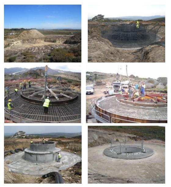
Photos 6.7 to 6.12 - Example of wind turbine tower foundation execution.
