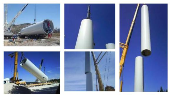
Photos 6.17 to 6.21 - Example of wind turbine tower assembly
