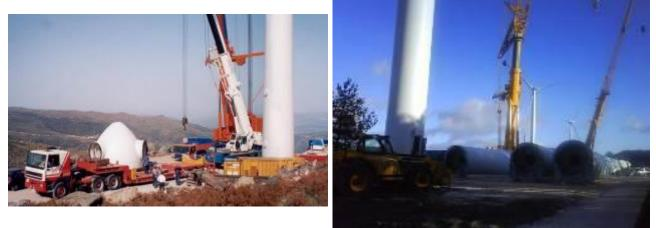
Photos 6.15 to 6.16 - Example of occupying a platform for wind turbine assembly.
